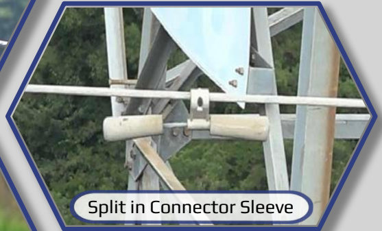
Split in Connector Sleeve
